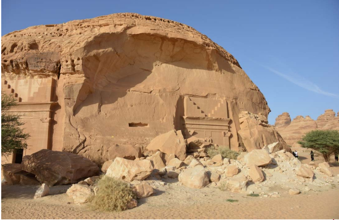
Hegra - Thermal stress, erosion and geomorphological instability process in KSA © Spizzichino
