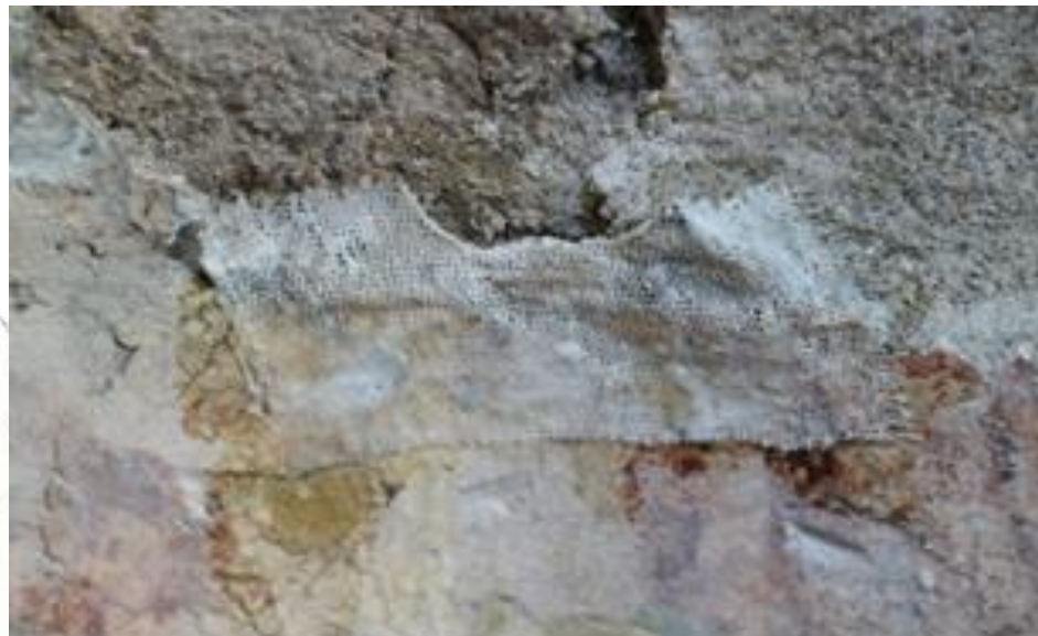
Temporary facing to avoid the falling of detached parts
