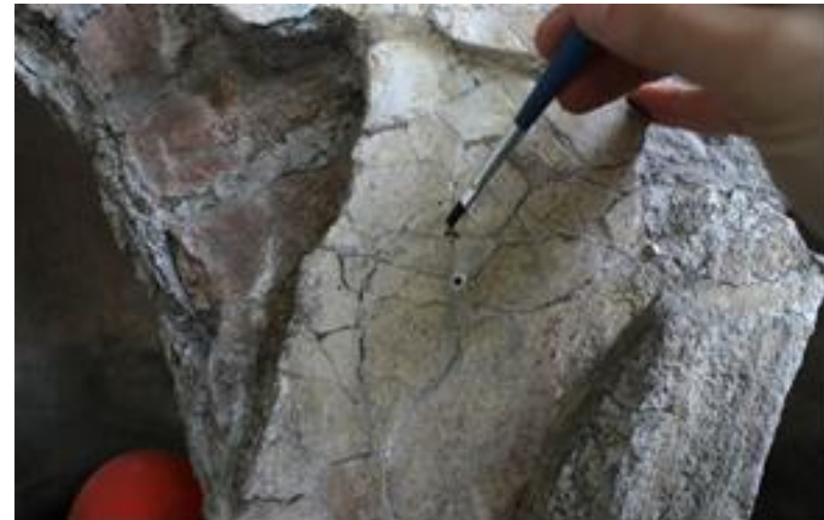
Temporary seals for mortar infiltration
