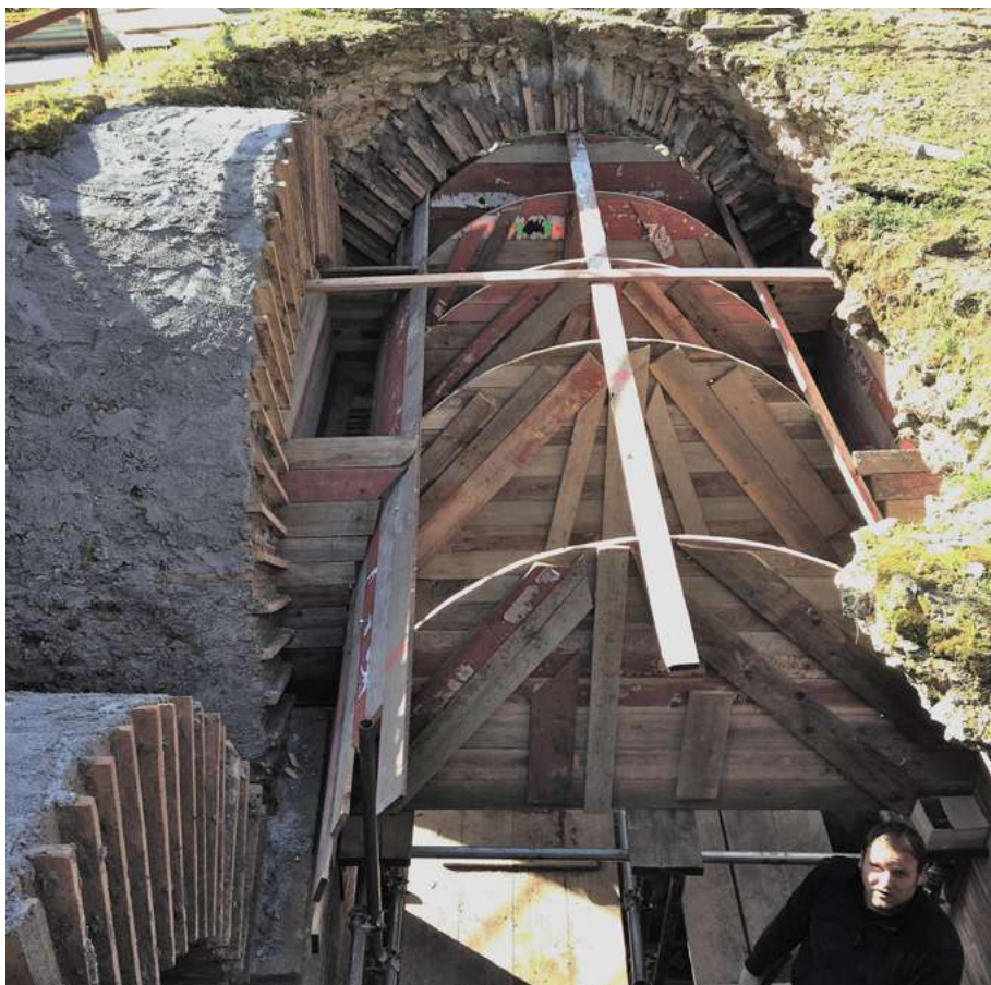
Fig. 7 The so-called Tomb of Gallienus. Reconstruction of the vaults and seismic improvement restoration works, carried out by Ettore Palmucci. Project by M.G. Filetici and C. Baggio, 2016 (Photo: S. Belotti 2017)
