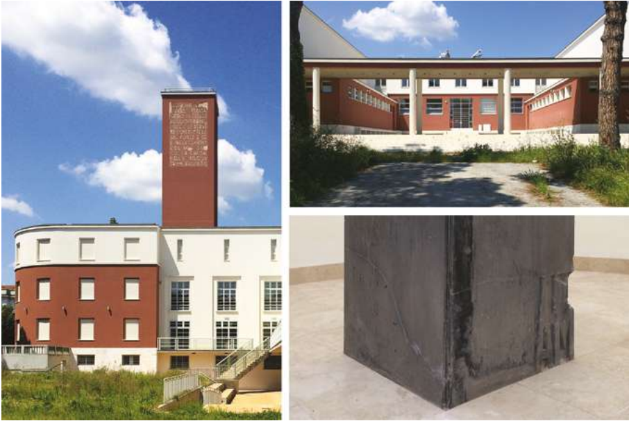
Fig. 3 C. Valle, Casa del Balilla, Forlì. The building as it appeared after restoration (Photos: G. Favaretto 2016)
