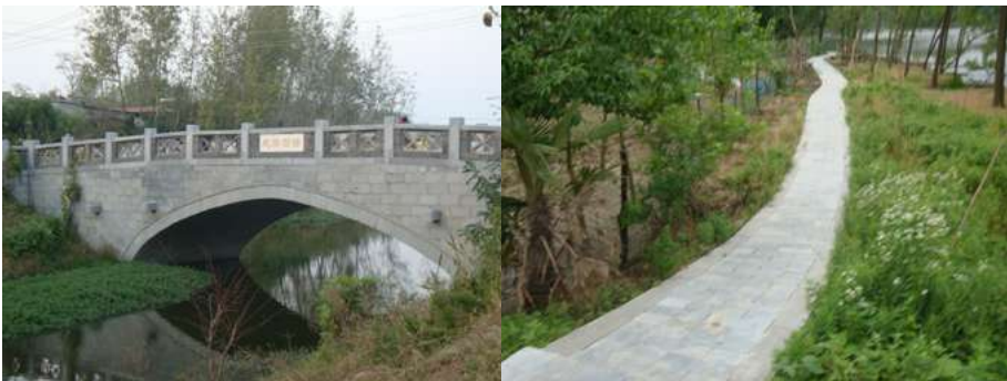
Fig. 5 Environment improvement of the canal
