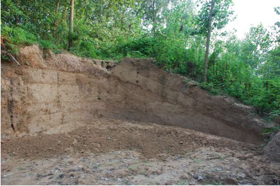
Fig. 1 A cross-section of the dyke at the west bank of the Inner Canal at Qingkou Complex, Huai'an, Jiangsu Province (Photo by the author 2008)
