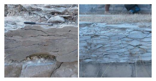
Fig. 1 Lath-shaped cracks in Chengde Mountain Resort
