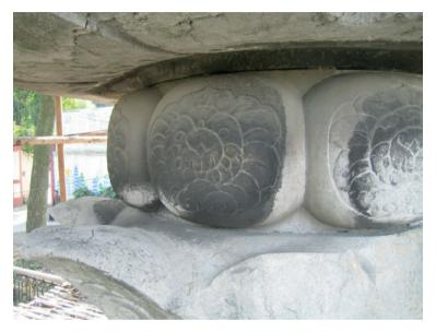
Fig. 2 Black deposition shell on the surface
