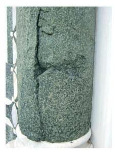
Fig. 5 Weathering phenomena in a serpentinite column
