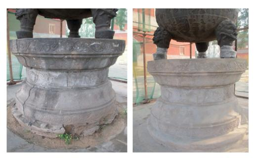
Fig. 4 Burner stone in Anyuan temple before and after repair
