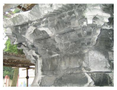
Fig. 3 Black deposition shell on the surface of brackets
