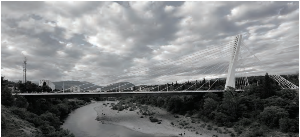
Fig. 2 The Millennium Bridge at Podgorica, Montenegro (photo by Ivan Laković).
